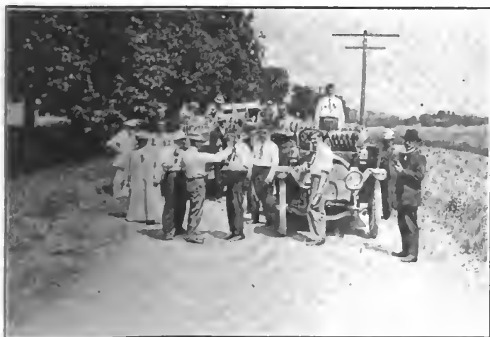
Inspecting McClintock's Cube Block Pavement near Charlotte
